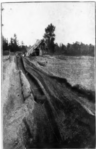
Operating \frac{1}{2} cu. yd. dragline scraper in sand and gravel pit.
